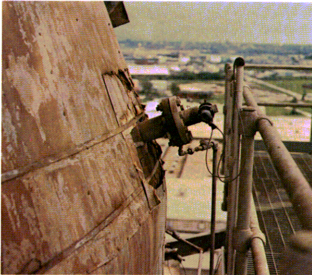
The K-1000 has no moving parts and can be serviced while the digester is under pressure.
